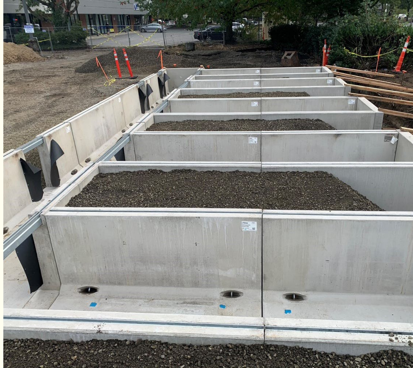
Pre-cast concrete trenches during construction
