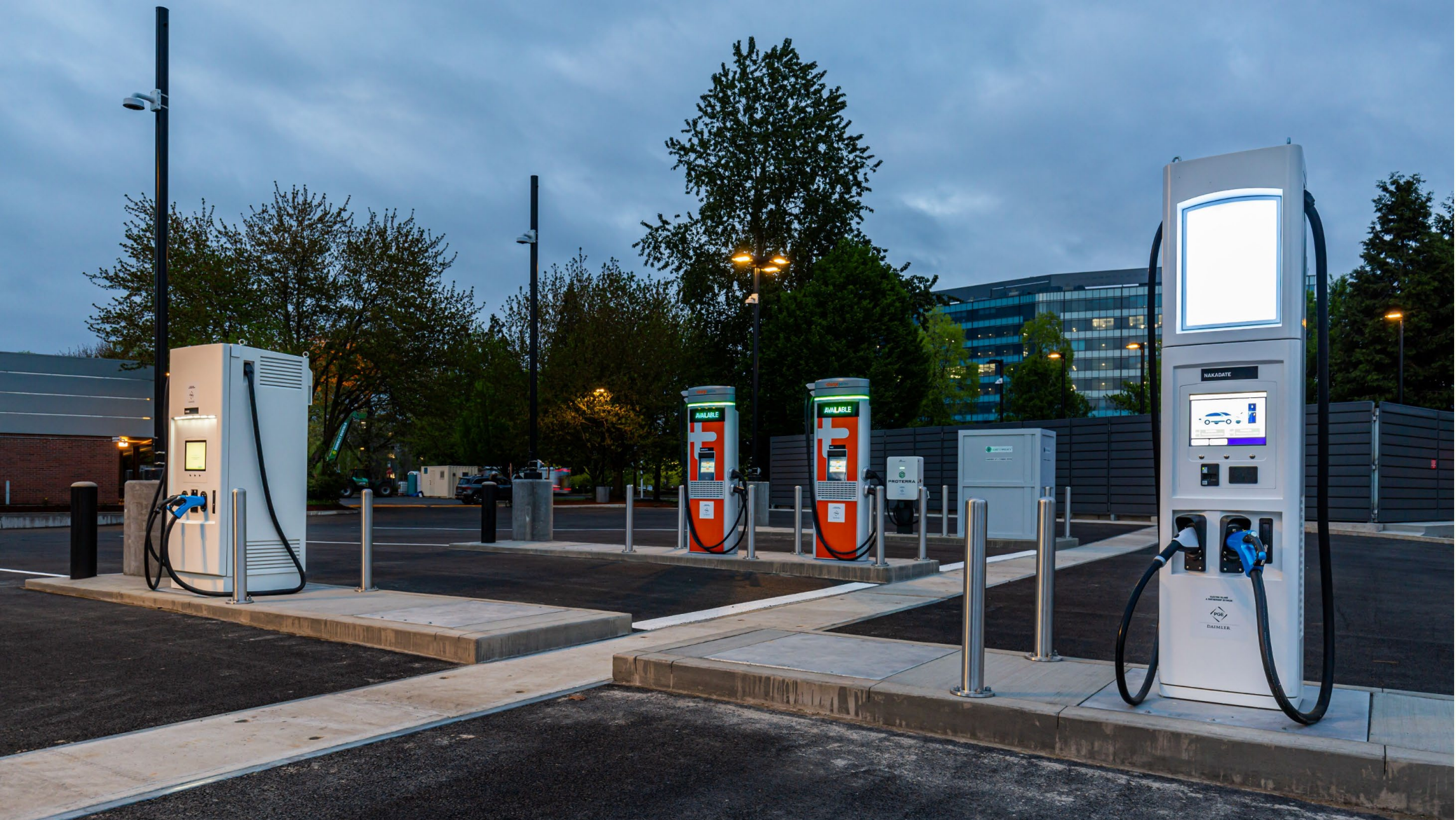
Finished site - note the extra bollards to prevent any accidents during truck maneuvering
