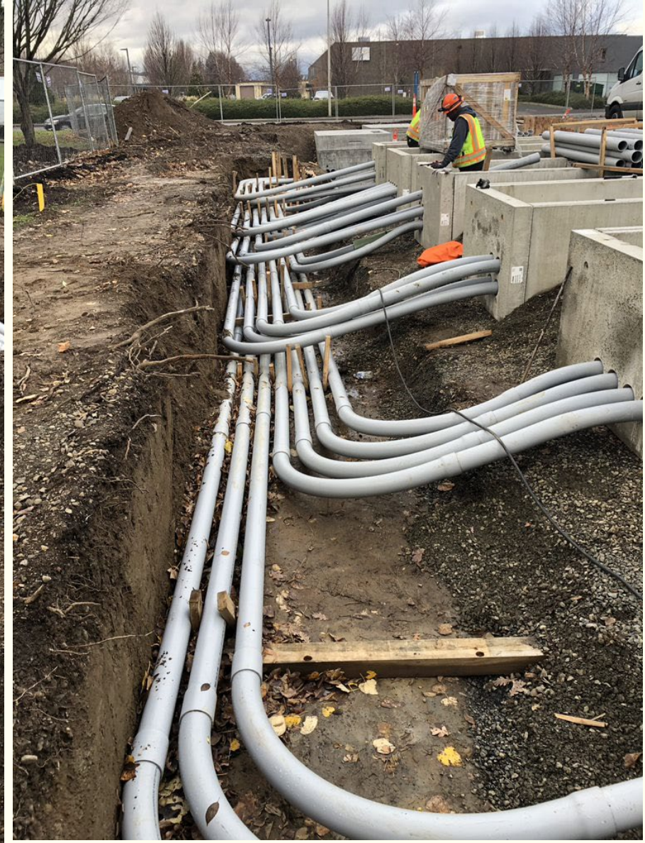
Tons of conduit! (for long-term electrical capacity)
