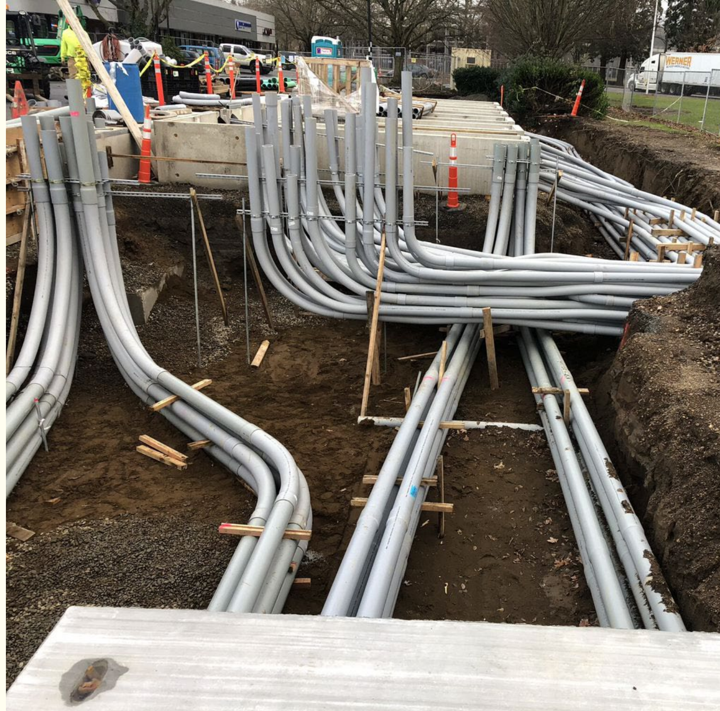
Tons of conduit! (for long-term electrical capacity)
